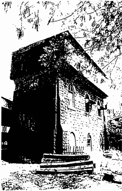
STRUCTURE WITHIN THANE RAILWAY STATION
