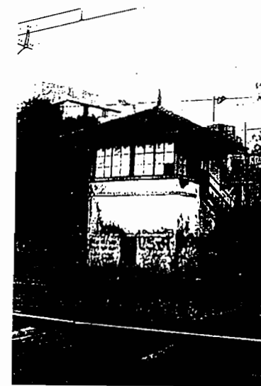
STRUCTURE WITHIN THANE RAILWAY STATION
